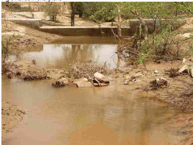
Fig-7 Masonry barrier across the stream
