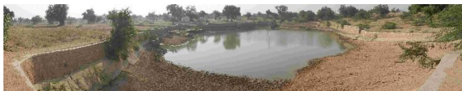
Fig-3 Improved Nadi with LDPE lining
