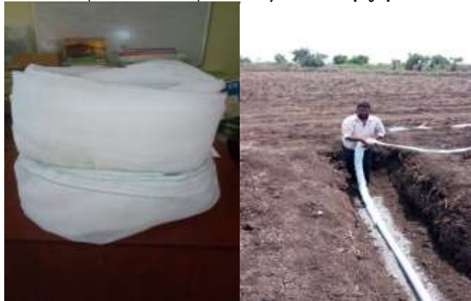
(a) Stitched nylon mesh (b) Wrapping nylon mesh to lateral pipe Fig-6 Envelope material
