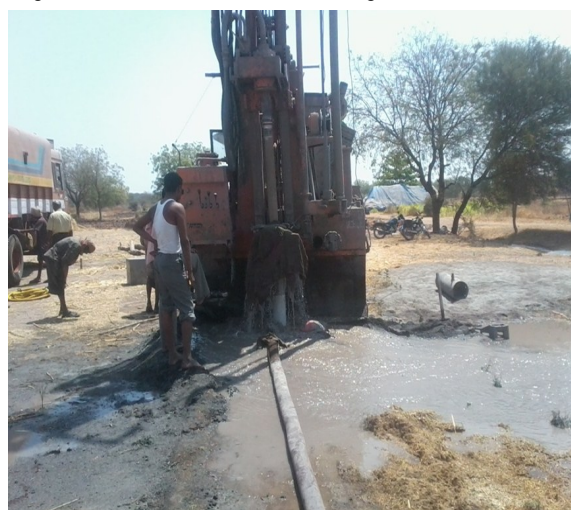
Fig. 4- Water coming out of bore well at the time of drilling
