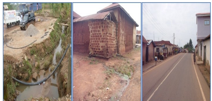
Fig. 2- Photos of parts of Akropong Township
