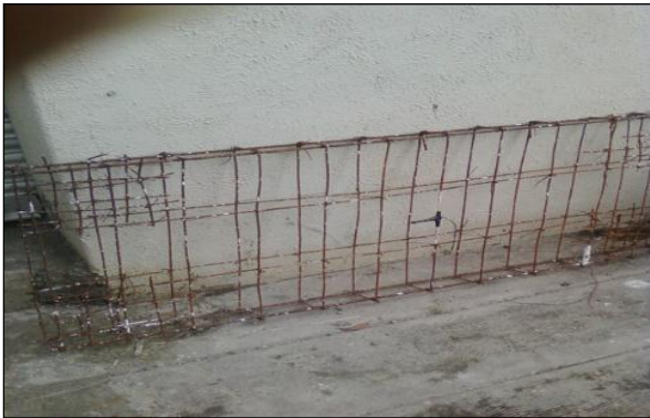
Fig. 3: Reinforcement Mesh of Simply Supported Deep Beam
