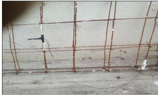
Fig.4: Reinforcement Mesh with Strain Gauges
