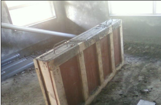
Fig.5: Casting Work of Simply Supported Deep Beam
