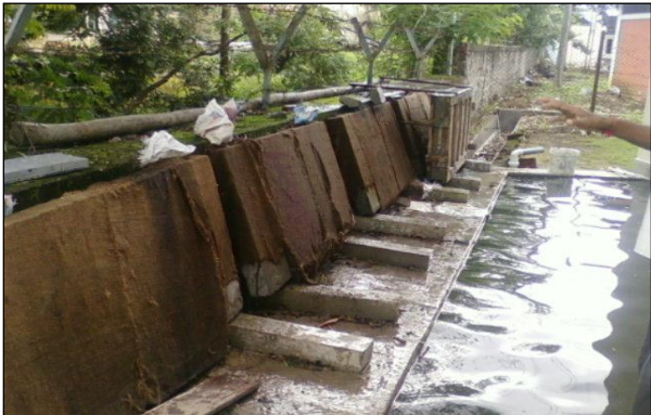
Fig.6: Curing Work of Simply Supported Deep Beam
